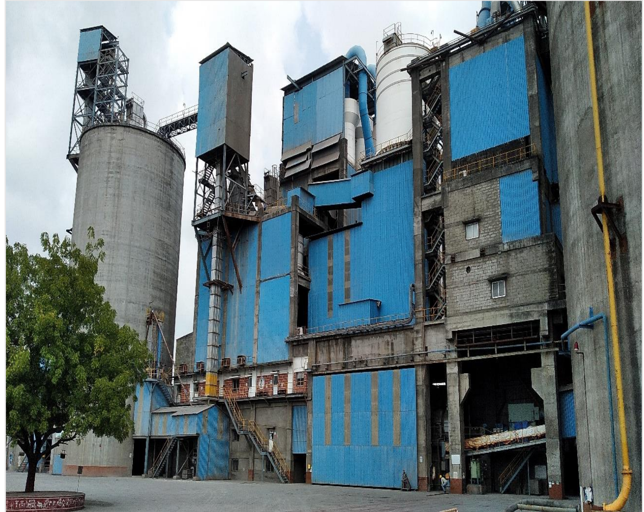
JK Lakshmi Cement Limited, Surat
